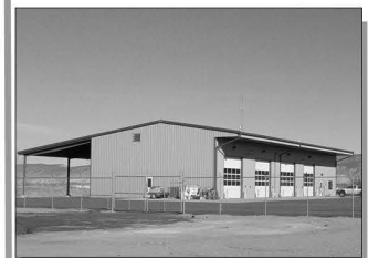
The new Olathe Public Works shop.
